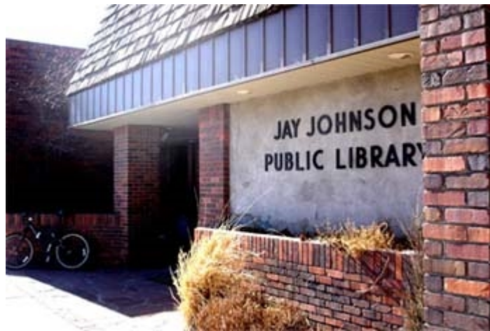
Jay Johnson Public Library shows off its new look - Quinter, KS. (Photo courtesy Jay Johnson Public Library)
